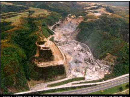
Figure 6. Belmont Quarry, Lower Hutt produces greywacke aggregate, asphalt and ready mix concrete. Photo: Winstone Aggregates Ltd.
