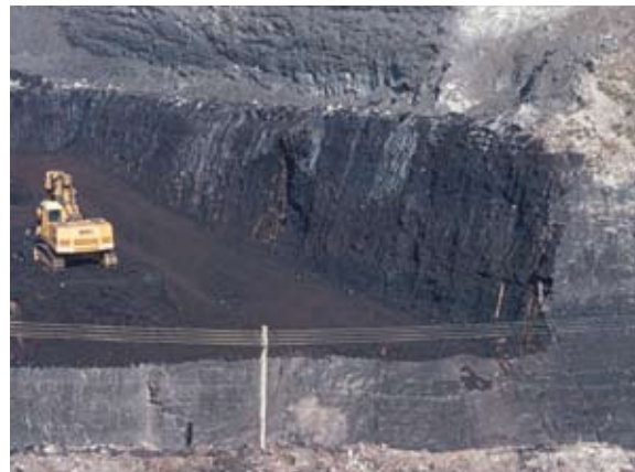
Mining a lignite seam up to 17.5 m thick, Waimumu, Eastern Southland. Photo: M Isaac
